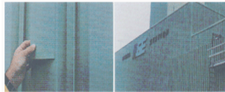
Ginna Nuclear Power Station, built in 1967, used PVDF coating and keep integrity of the coating for near 40 years.
